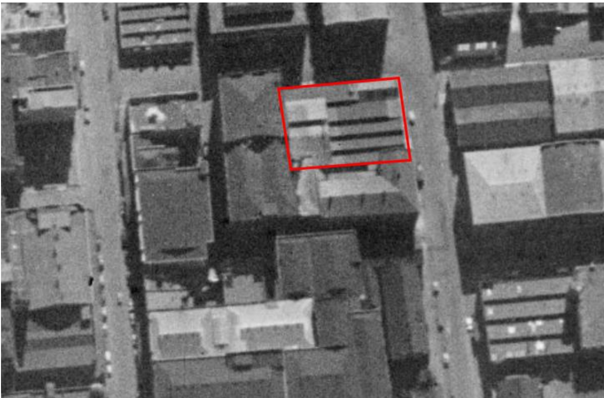
Figure 18 – Aerial photograph dated to c.1943. Approximate location of the subject area as indicated in red.
